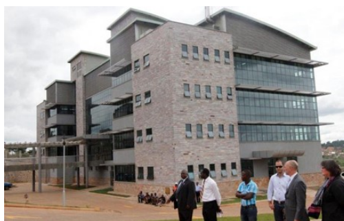
The new CPHL Building in Butabika.
